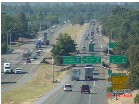
Interstate 5 was designed to accommodate a third vehicle lane in either direction within the existing median.
